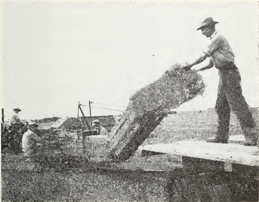
FIGURE 17.—Loading trailed wagon directly from baler. It is estimated that trailing a wagon as is done here reduces baling speed about 15 percent but it eliminates the strenuous labor of lifting bales from ground onto wagon.
